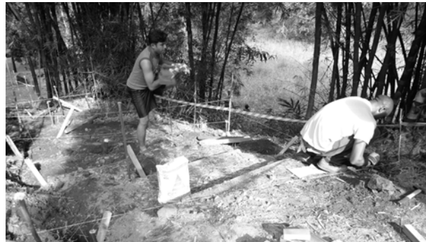
Figure 6 - Building of the scale 1 model Threshold loft To build the full scale model of the Threshold loft, students transformed the natural slope of the site to create a succession of levels and thus literally inhabit the topography. Courtesy: René Paul Savignan.
