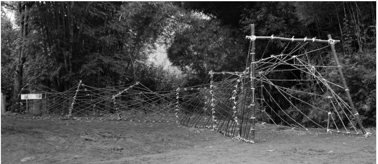
Figure 10 - The Link One portion of the full scale model of the covered path connecting all the rooms together called the Link by the students using bamboo structure. Courtesy: René Paul Savignan.
