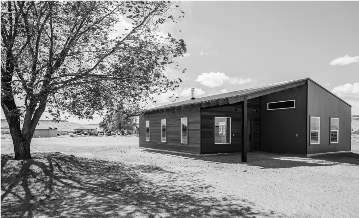
Figure 1: Lone Tree, completed by DesignBuildBLUFF students in the Spring of 2017. Courtesy: DesignBuildBLUFF.
