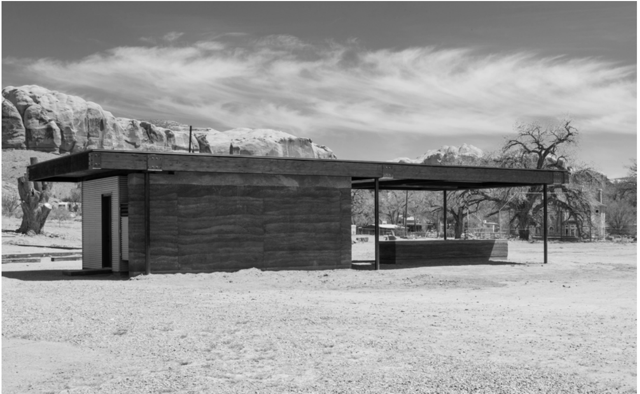
Figure 4: Fire Mesa, completed by DesignBuildBLUFF students in the Spring of 2018. Courtesy: DesignBuildBLUFF.
