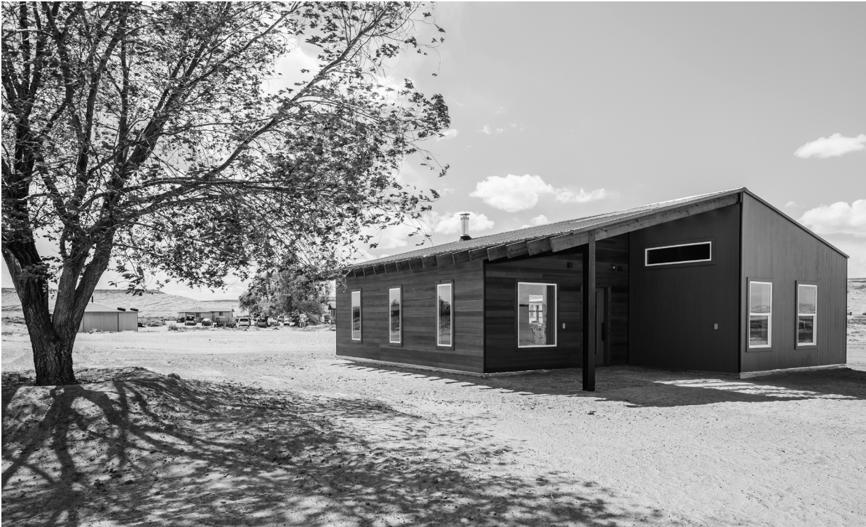
Figure 1: Lone Tree, completed by DesignBuildBLUFF students in the Spring of 2017. Courtesy: DesignBuildBLUFF.
