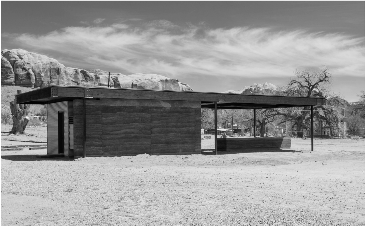
Figure 4: Fire Mesa, completed by DesignBuildBLUFF students in the Spring of 2018. Courtesy: DesignBuildBLUFF.
