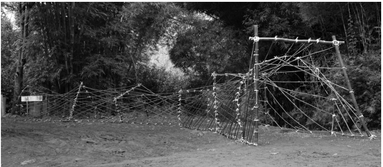
Figure 10 - The Link One portion of the full scale model of the covered path connecting all the rooms together called the Link by the students using bamboo structure. Courtesy: René Paul Savignan.
