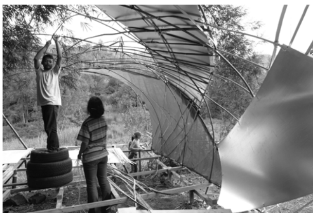
Figure 3 - Building of the scale 1 model - Gastronomica Students, during the one week of building, build a full scale model of their Gastronomica room using bamboo, prefabricated metal sheeting and green mesh shades. Courtesy: René Paul Savignan.
