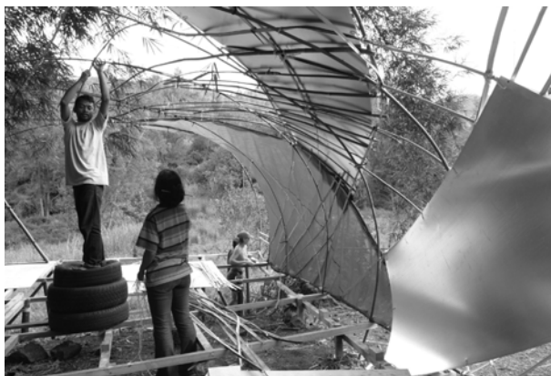
Figure 3 - Building of the scale 1 model - Gastronomica Students, during the one week of building, build a full scale model of their Gastronomica room using bamboo, prefabricated metal sheeting and green mesh shades. Courtesy: René Paul Savignan.
