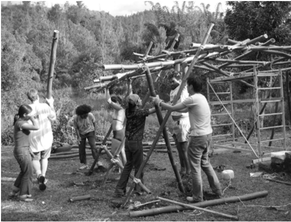
Figure 11 - Building of the scale 1 model - Possible Loft Students build the full scale model of Possible loft which is a large space free of pillars whose structure revisits a traditional Chinese structure assembled flatwise on the ground and then raised in the upright position with the force of only a few persons. Courtesy: René Paul Savignan.
