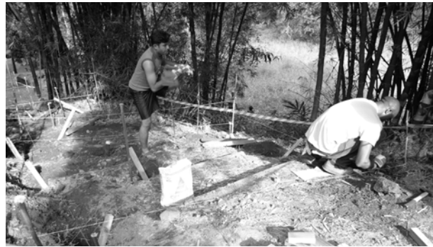
Figure 6 - Building of the scale 1 model Threshold loft To build the full scale model of the Threshold loft, students transformed the natural slope of the site to create a succession of levels and thus literally inhabit the topography. Courtesy: René Paul Savignan.
