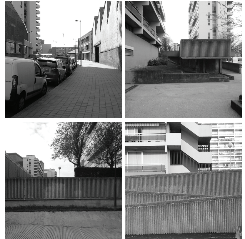
Figure 1(a-d): Avenue de l'Héliport, Social Housing and Plinth. Courtesy: The author, October 2018–August 2019
