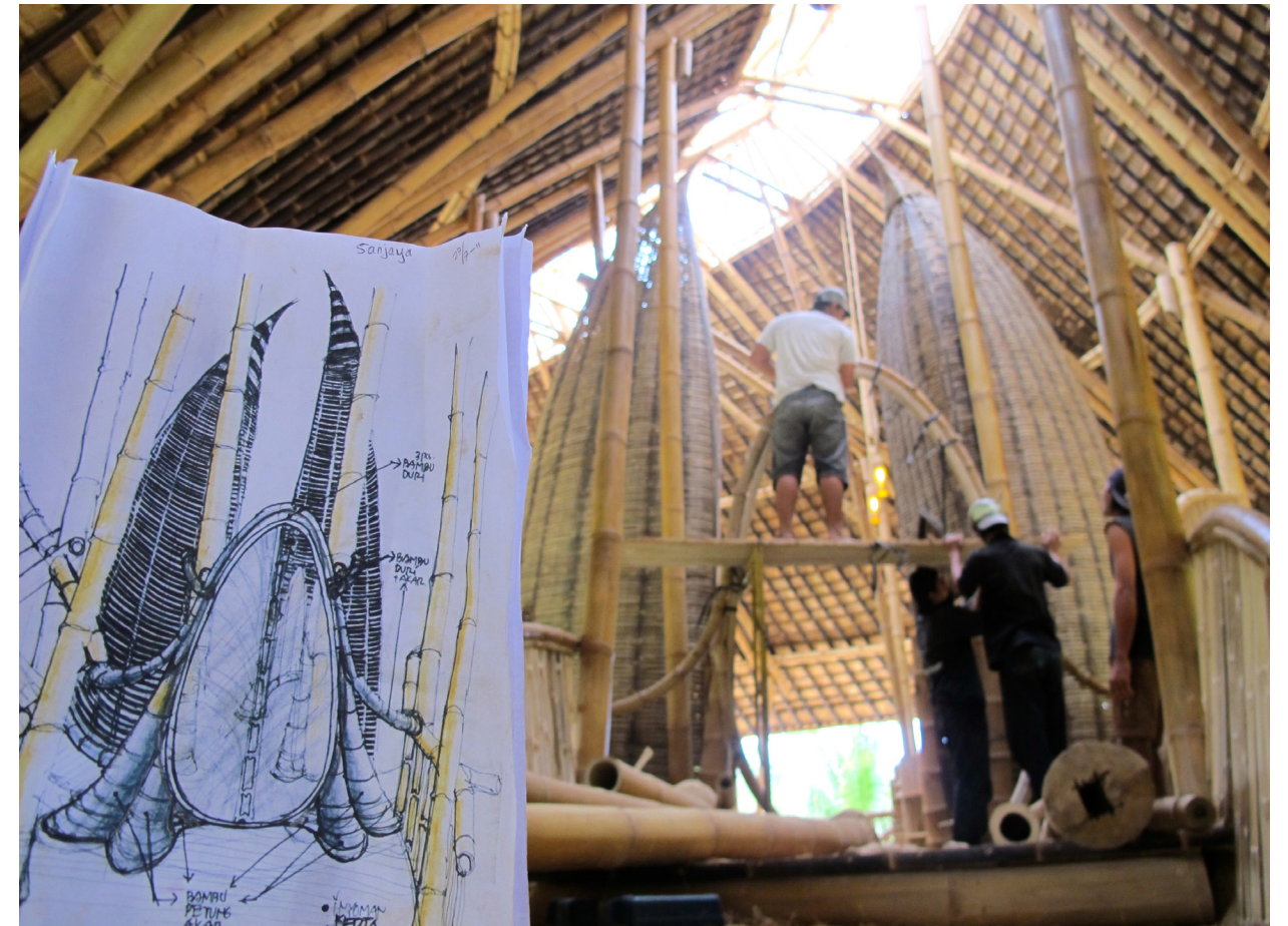
Figure 6: The design process moves from hand sketch to bamboo model to construction (©Ibuku) courtesy of Elora Hardy / Ibuku.
