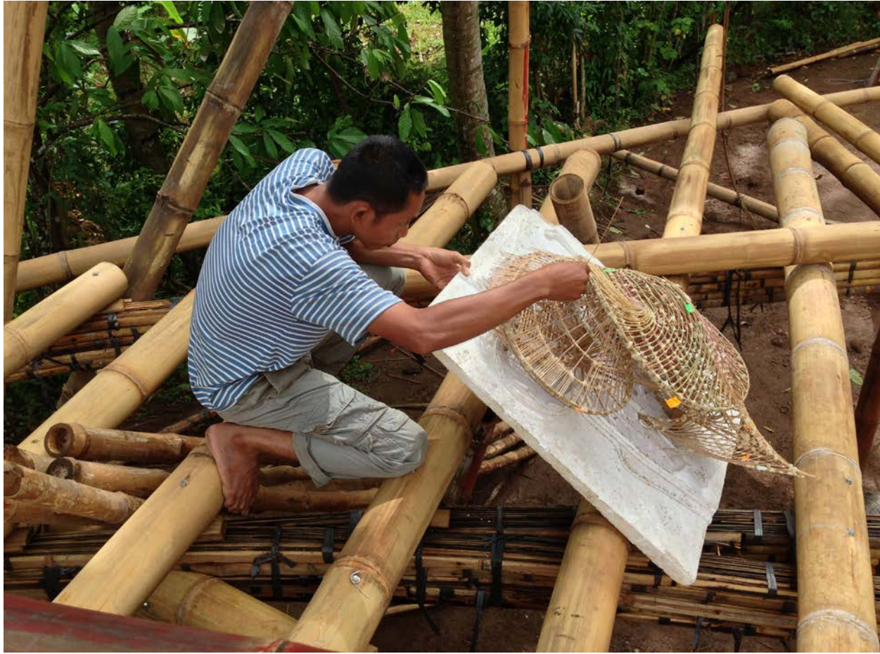
Figure 7: The construction is executed by scaling directly from the 1:50 model in the field (©Ibuku) courtesy of Elora Hardy / Ibuku.
